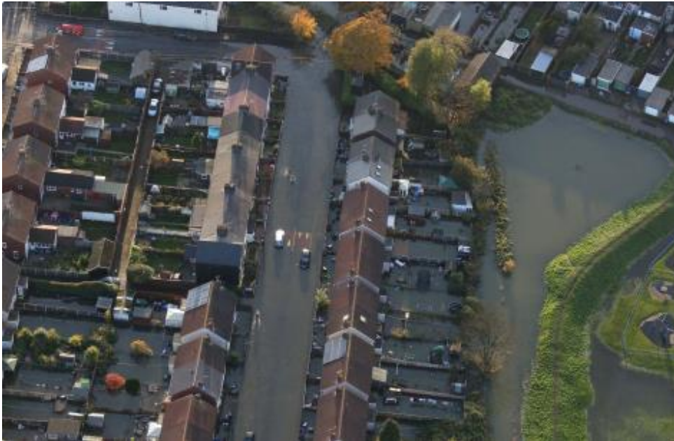
Figure 7. Flooding at Bentley during the 2019 flood event.
